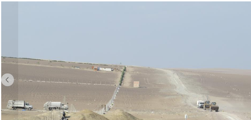
RELLENO SANITARIO – ICA
